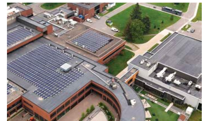
▲ Large-scale electric heat pump and thermal storage facility at Confederation College—the first of its kind in Northwestern Ontario.
