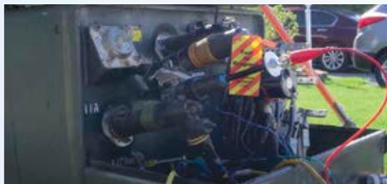
▲ Synergy North Cable Testing Activities
